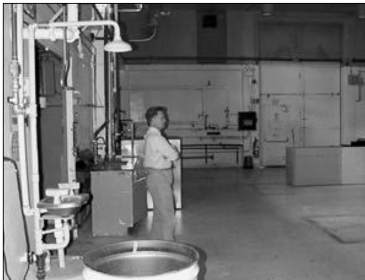
Chemical Science and Technology (CST) Division Director Alex Gancarz inspects a section of Building 2 in Technical Area 21 to make sure everything that needed to be removed from the site was indeed removed.
