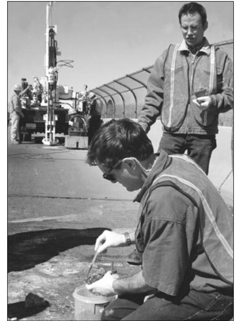
George Guthrie, kneeling, washes a concrete core taken from the Paseo del Norte overpass of Interstate 25 on Albuquerque's north side. The concrete cores were previously stained to test for alkali-silica reaction. Standing at right is Bill Carey. Photo by James E. Rickman
