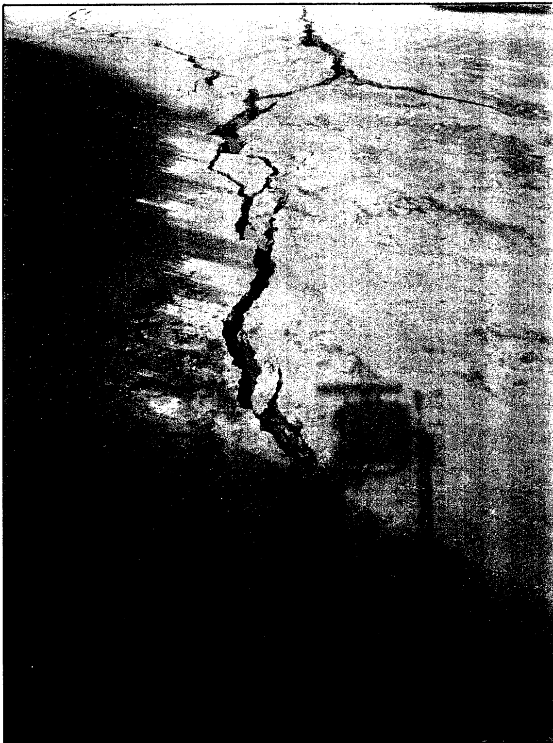
Figure 3-9. Cracks in prepared surface (trailer park) on Rainier Mesa. These cracks formed prior to collapse sink formation.
