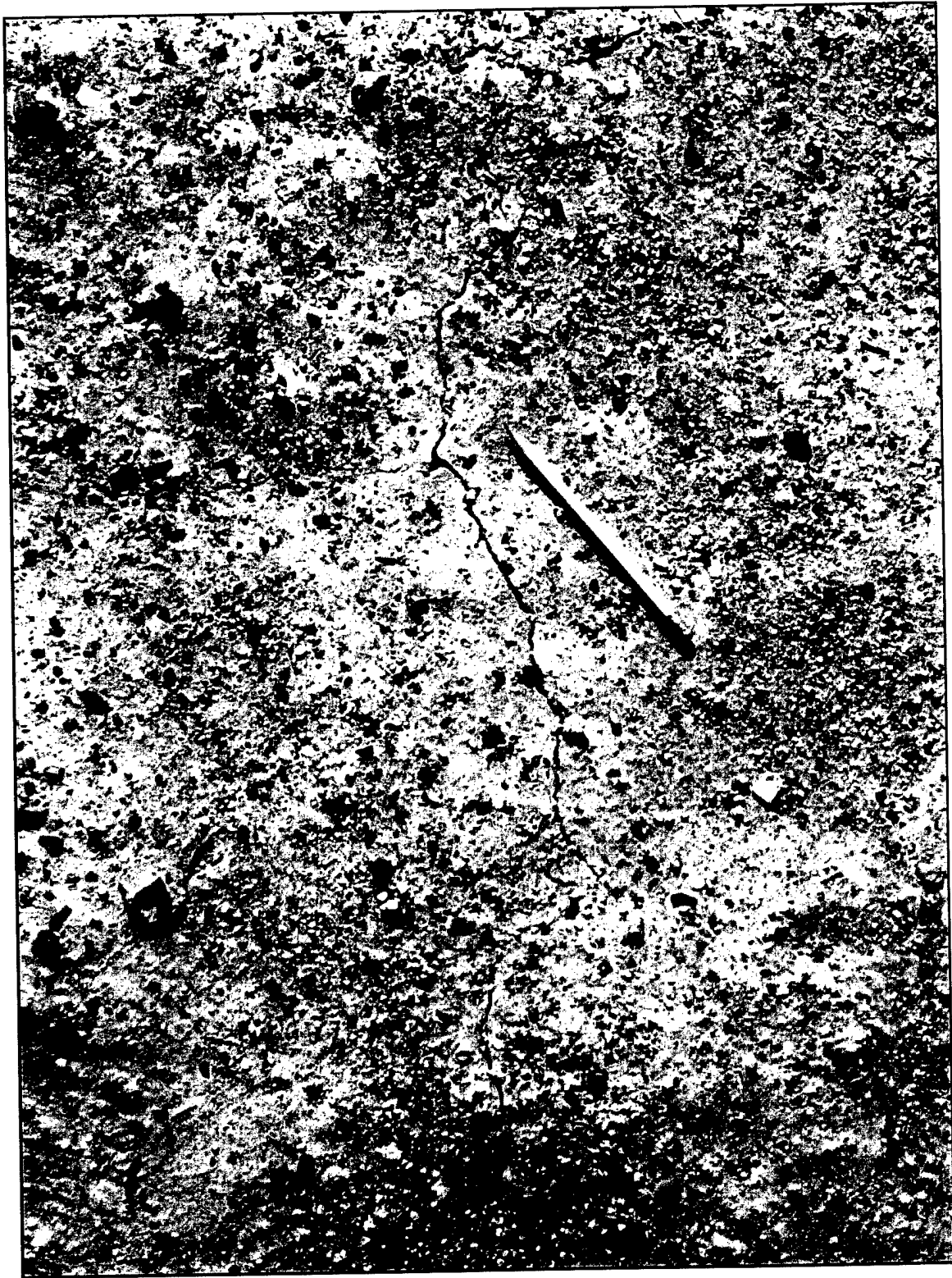
Figure 3-7. Hairline crack in alluvium resulting from the DALHART test (U4u).
