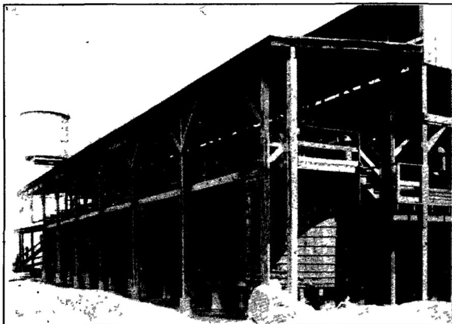
FIGURE 64. Boiling Tubs for Purification of Nitrocellulose.
